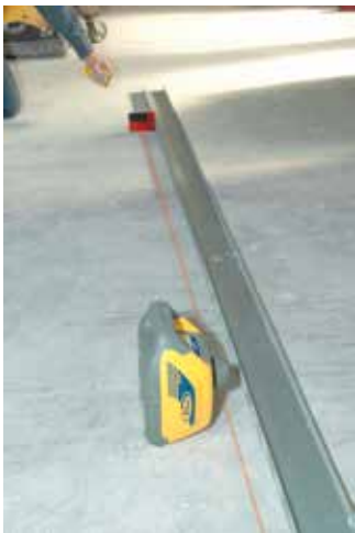
Vertical alignment application
