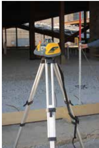
Exterior application setting forms
